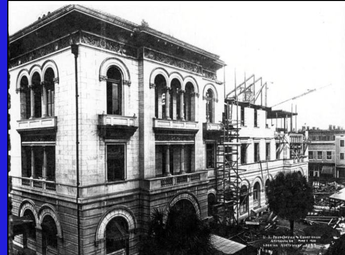
LOOKING NORTHWEST FROM THE CORNER OF W. YORK & BULL STREETS
