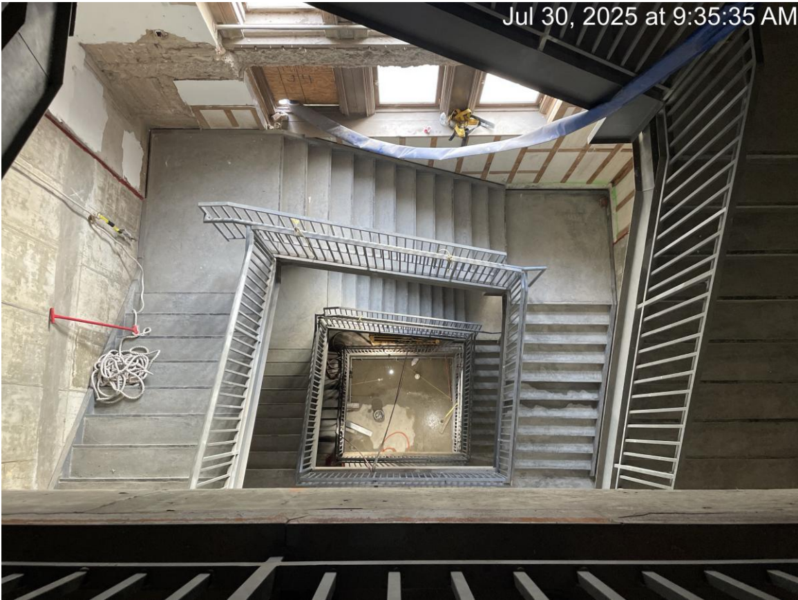
Floor 4 – Staircase #3 installation progress
