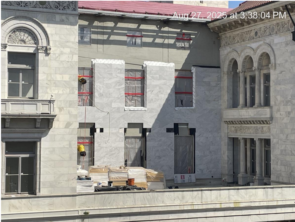
Bridge Connector ongoing façade installation
