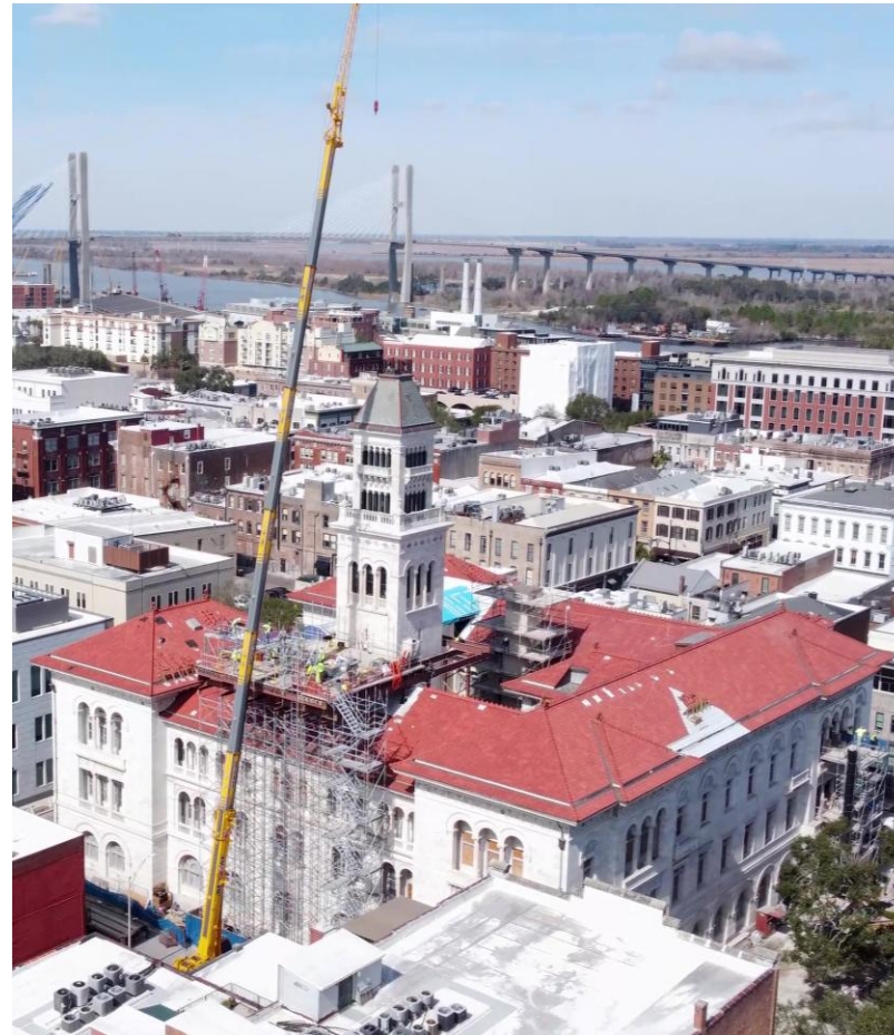
Tower w/ Structural and Architectural Upgrades
