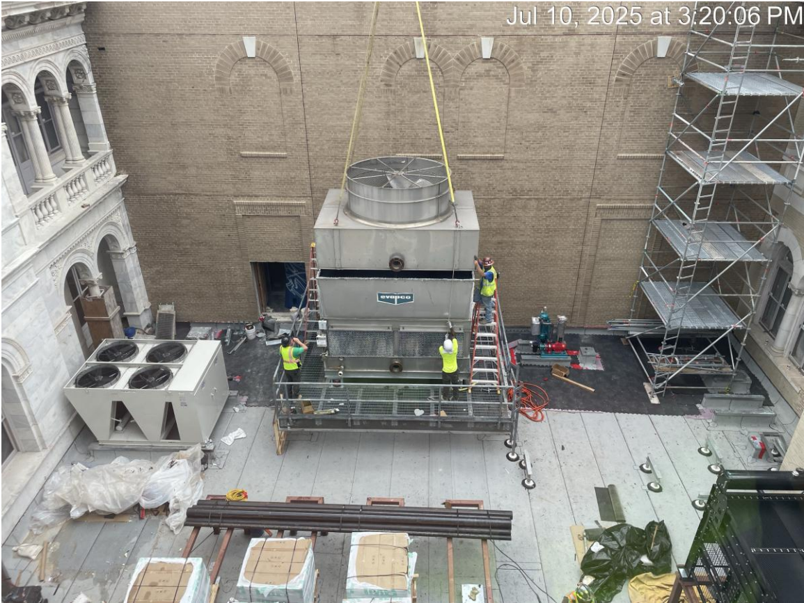
Floor 2 (Lightcourt) – Cooling Tower installation progress
