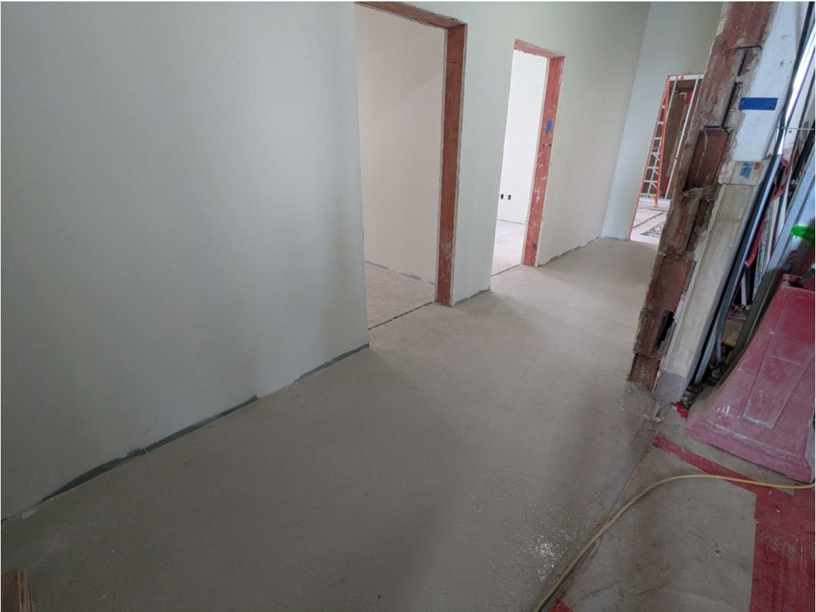
Floor 1 & 3 – Terrazzo installation progress
