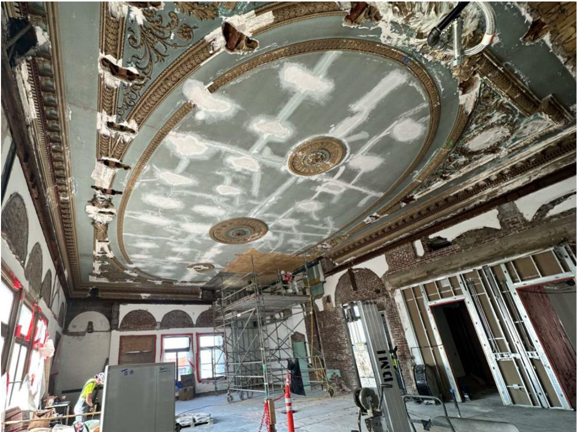
Jury Assembly – Historic Ceiling Plaster progress
