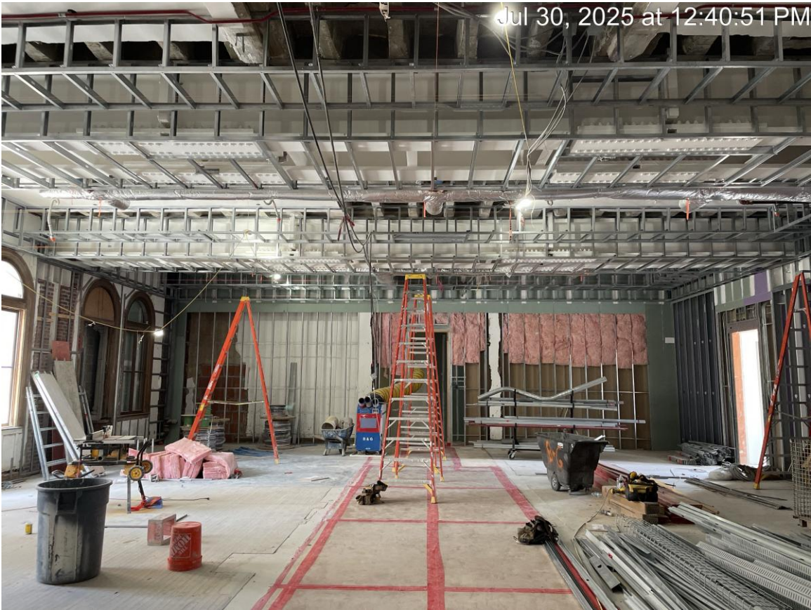
Floor 2 Sr. District Courtroom –Soffit framing installation progress
