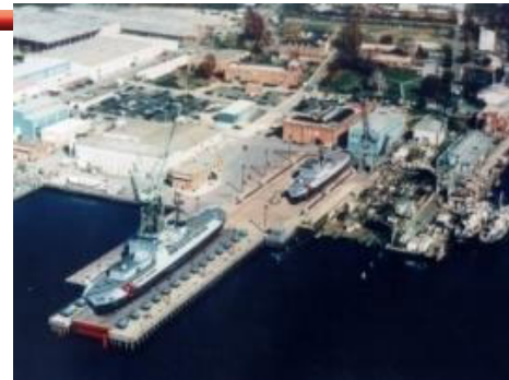
Industrial Facilities & Bases
