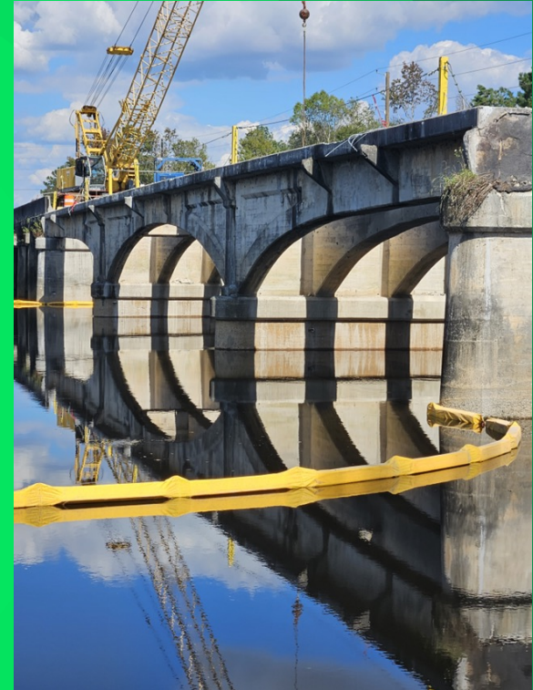
Stage One Demolition
