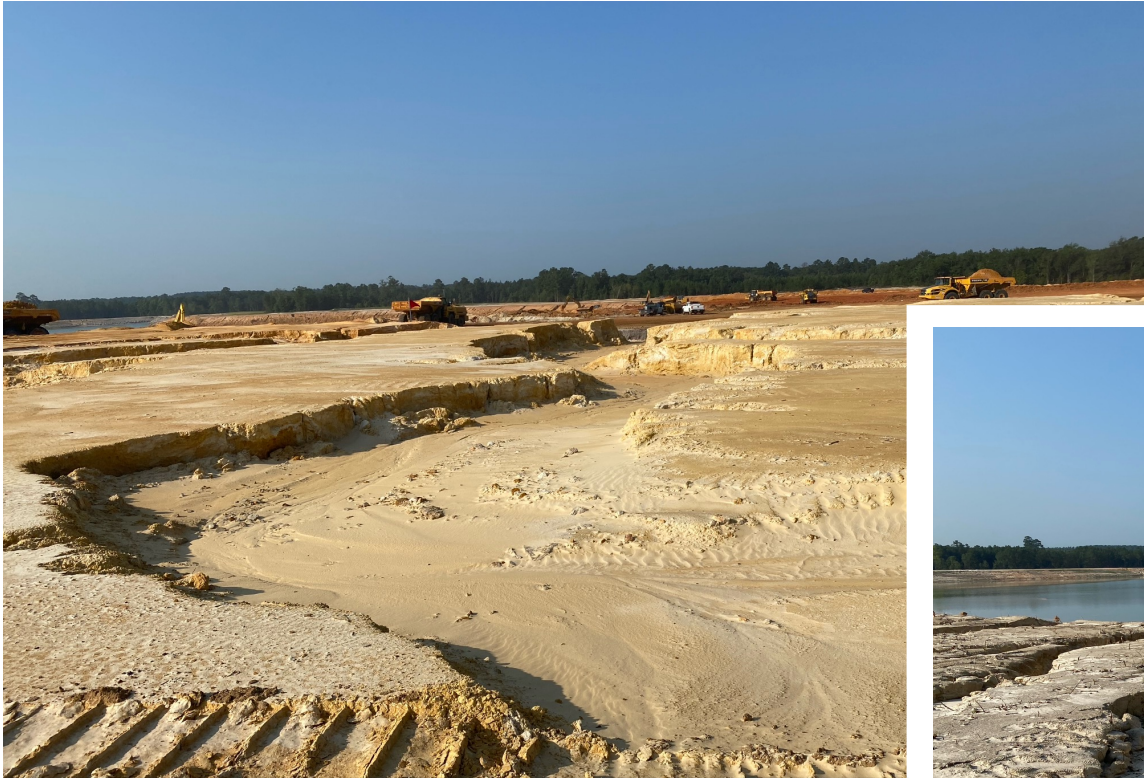
Sandy Soil Severe erosion
