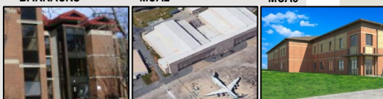
FT STEWART VOLAR BARRACKS ROBINS AFB PAINT/DE-PAINT HANGAR ROBINS AFB ABMS OPS FAC.
