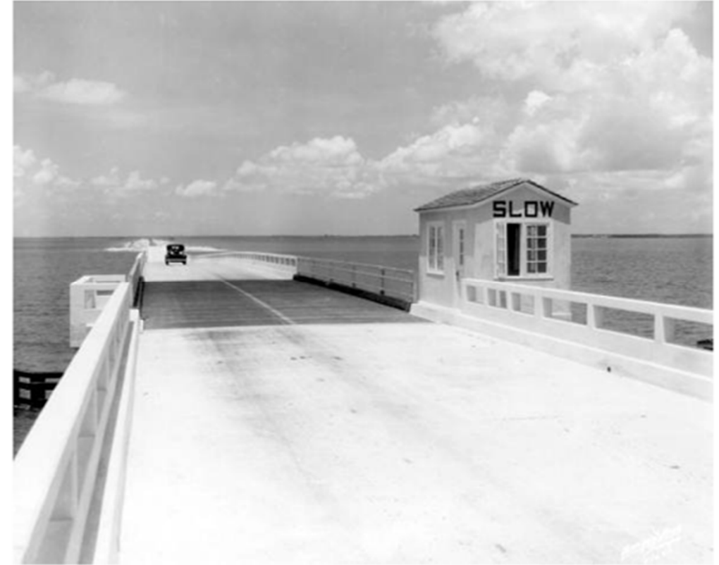
Historic Photo of Courtney Campbell Causeway (1934)
