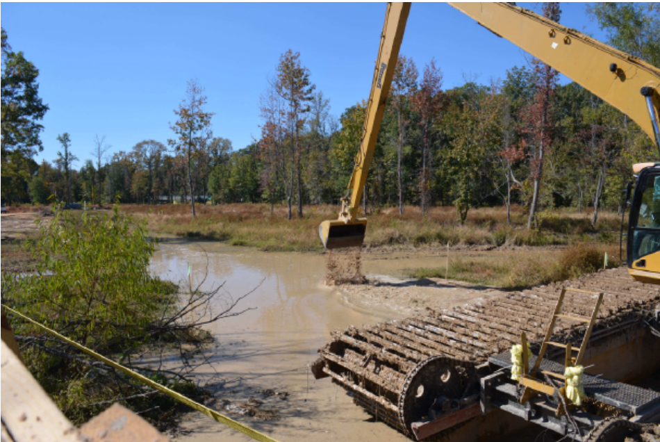
Reactive Cap Placement in Open Water Area
