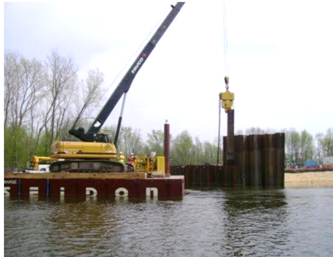
Physical Barriers to Control and Contain Disturbed Soils and Sediments
