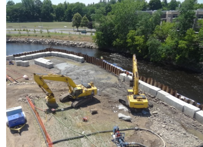
Removal with River Bypass
