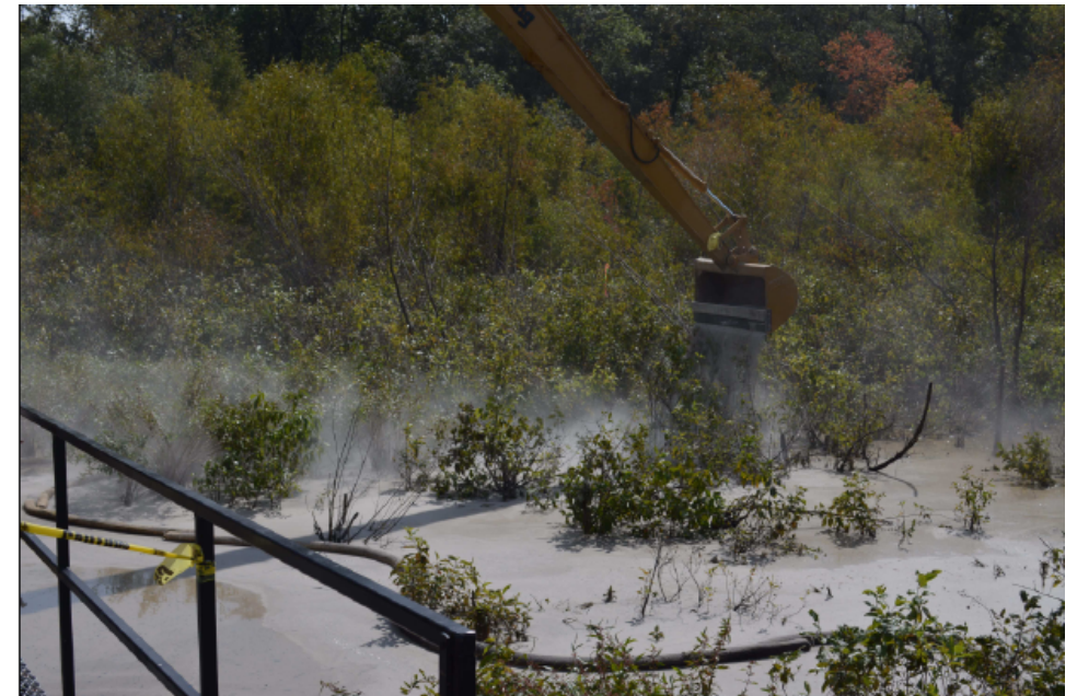
Amendment Placement over Heavily Vegetated Area
