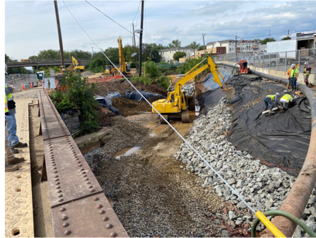
Removal With Pump Around Stream Flow
