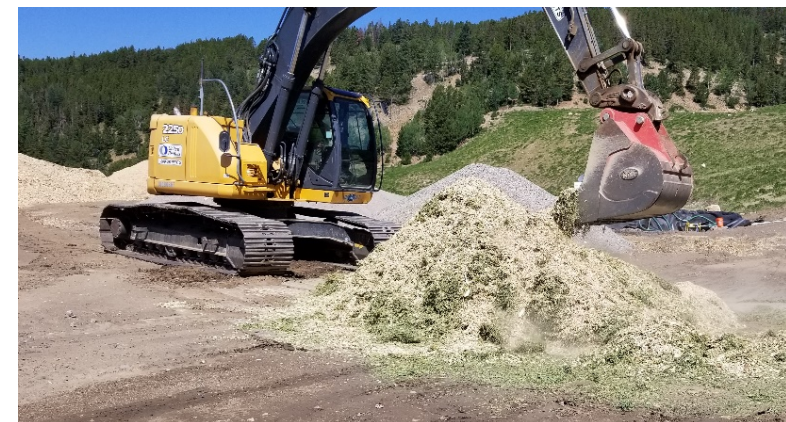
Mixing of Biochemical Reactor Media for Placement into Cells
