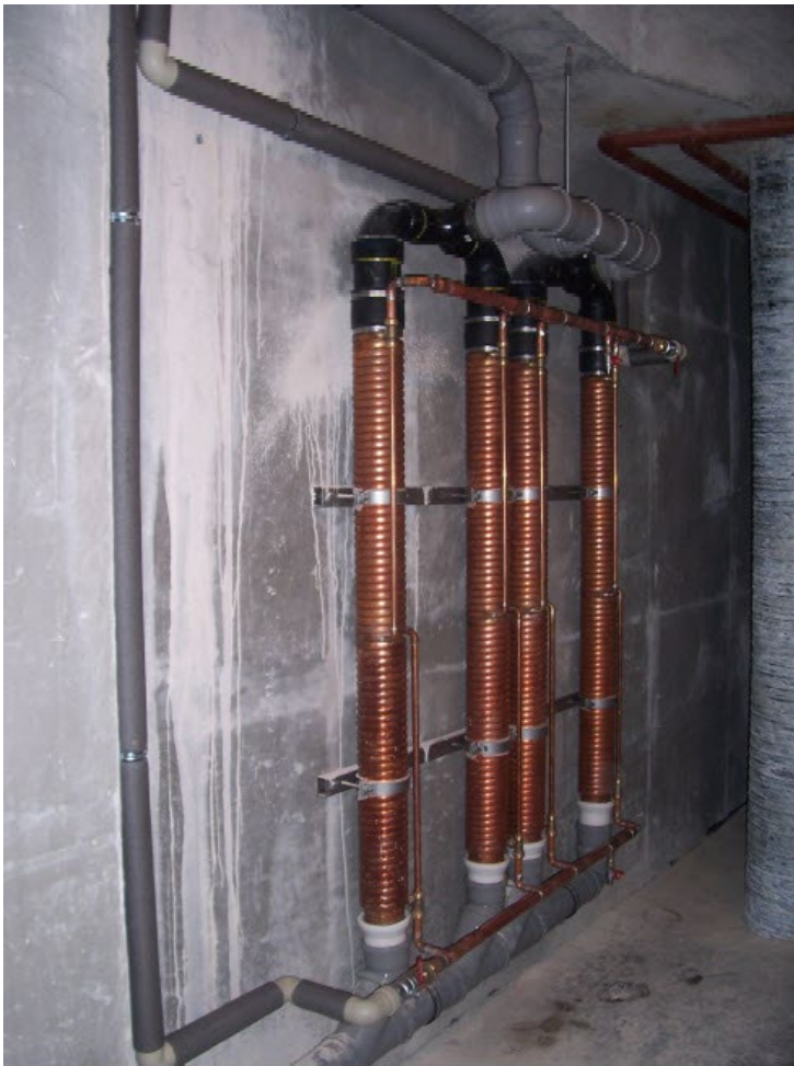
Gravity film heat exchangers save 34% on domestic hot water heating energy
