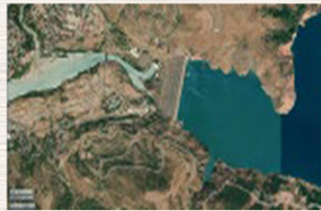
Dam Inspection - Uzbekistan
